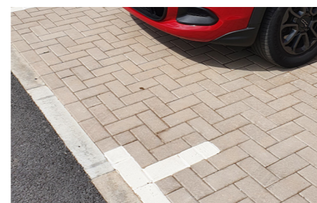
PCC block paving - parking bays
